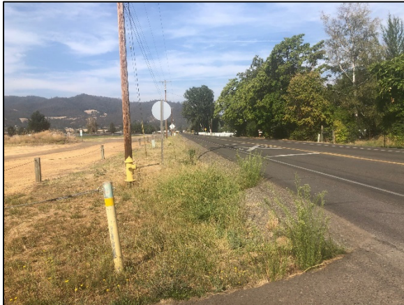
From maintenance access, looking west
