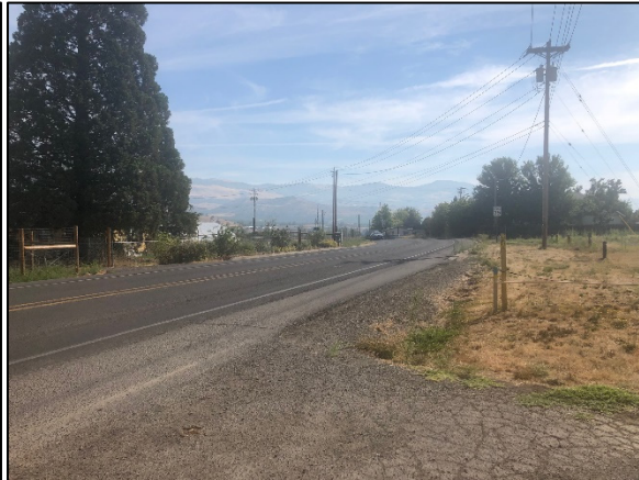
From maintenance access, looking east
