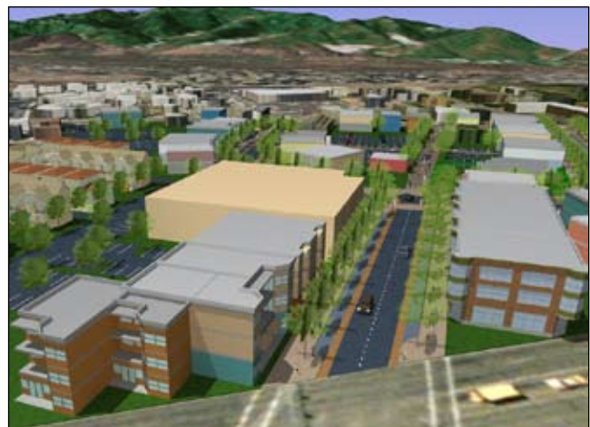
Intersection of Highway 99 and West Valley View looking west.
