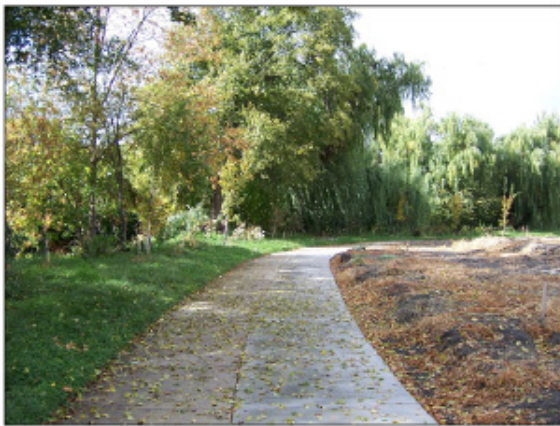
CONCRETE TRAIL (EXISTING SECTION OF WAGNER CREEK TRAIL)
