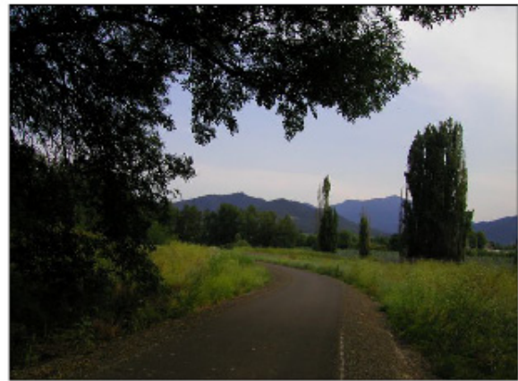
ASPHALT TRAIL (EXISTING SECTION OF BEAR CREEK TRAIL)
