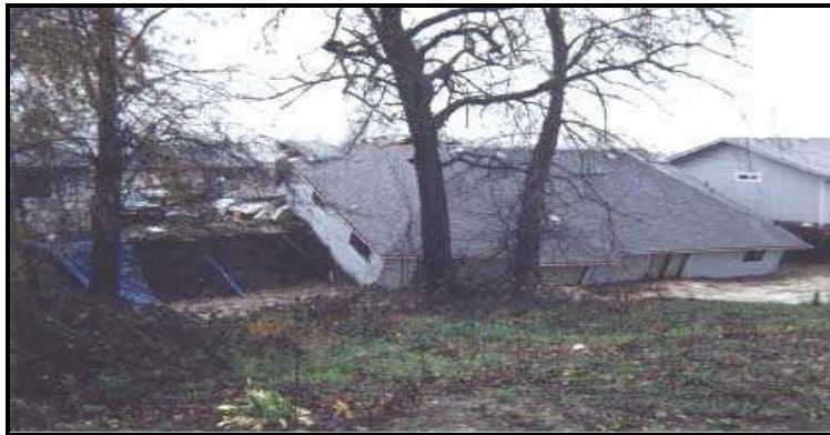
Figure 2: Photo of 265 Joseph Drive during the Flood of 1997
