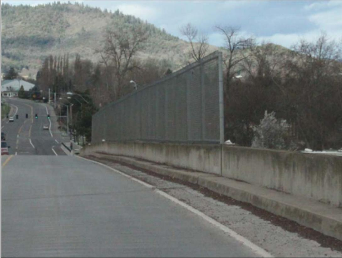
**Figure 8b. Sample Retrofitted Bridge Rail**
