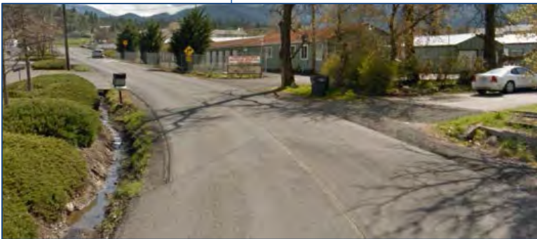
No Curb, Gutter, or Sidewalk
