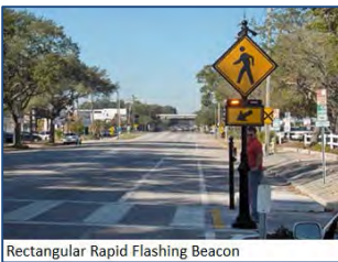
Rectangular Rapid Flashing Beacon
